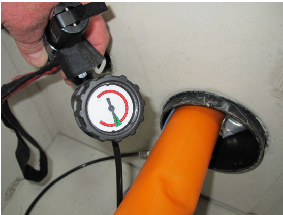
Filling and sealing the TE connectivity ADE / TDUX
