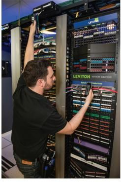
Reading FiberChek probe results on a smartphone
