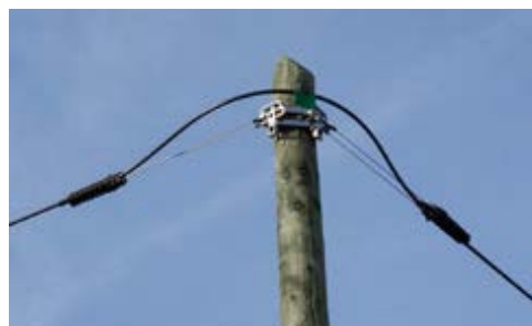
Left : single dead-end; Right :double dead-end
